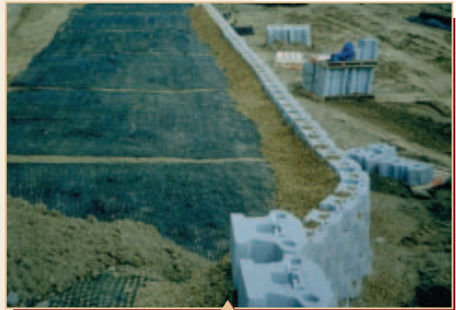
Keystone Compac units installed with geogrid.
