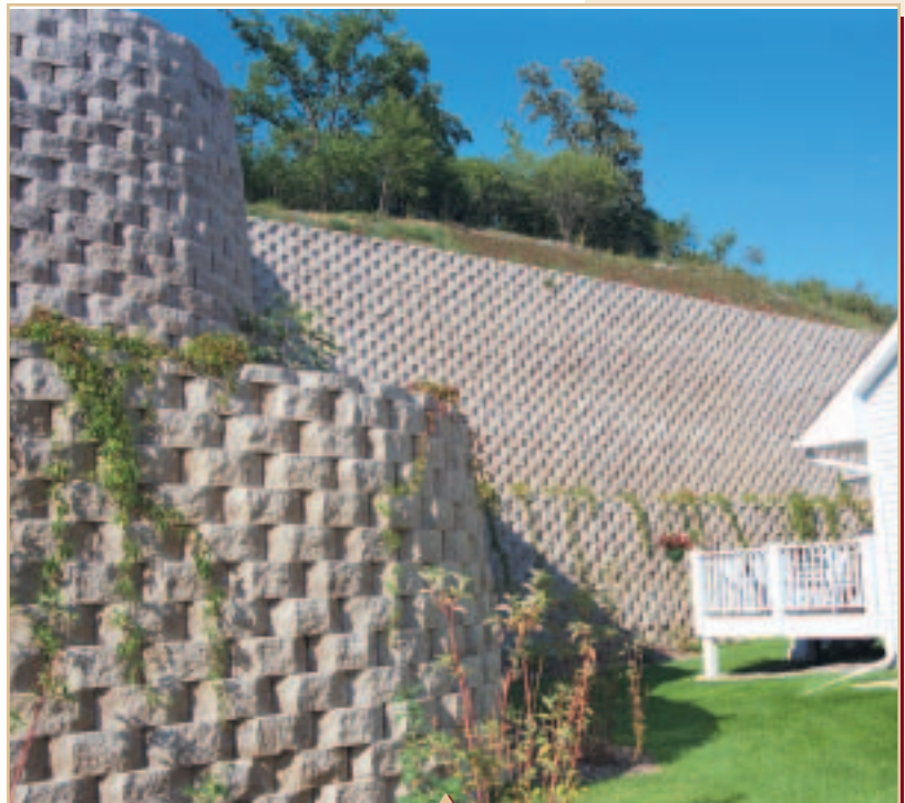
30' (9m) high Keystone Wall in Edina, Minnesota creates space for housing development
