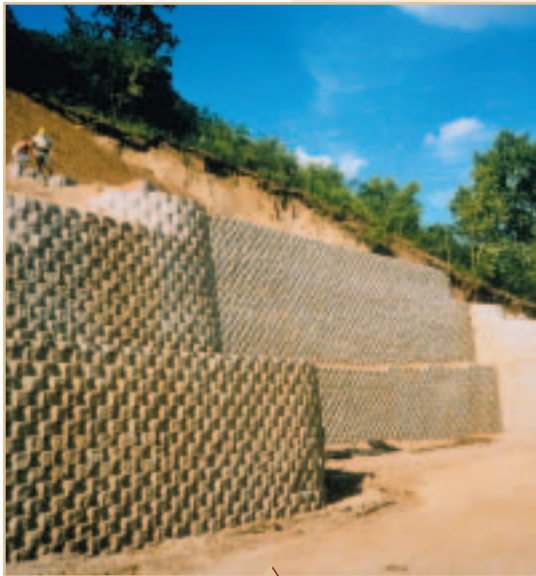
30 foot high terraced Keystone wall with a sloped top elevation.
