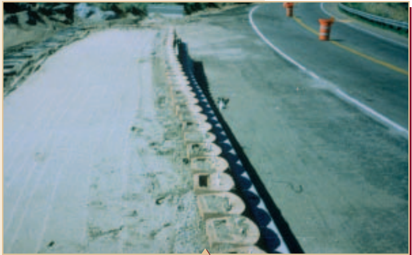
Falling rock barrier - Keystone wall facing the road, with reinforced soil zone behind, backed by wall of old tires.
