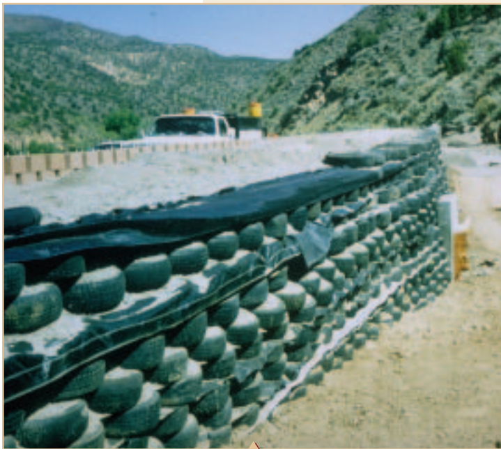
Tire wall at back of the barrier, cushions falling rocks and directs them into the catchment area.
