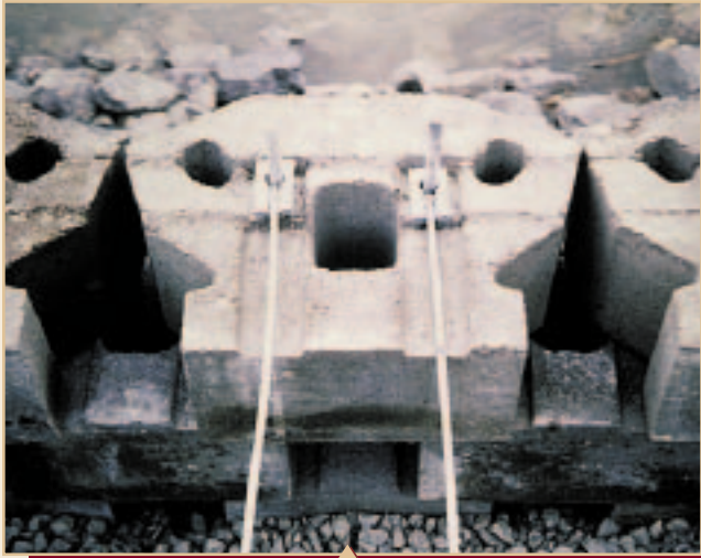
Detail of Keystone Unit & Keystrip Reinforcement
