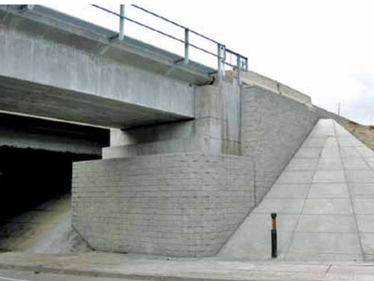
Completed Abutment
