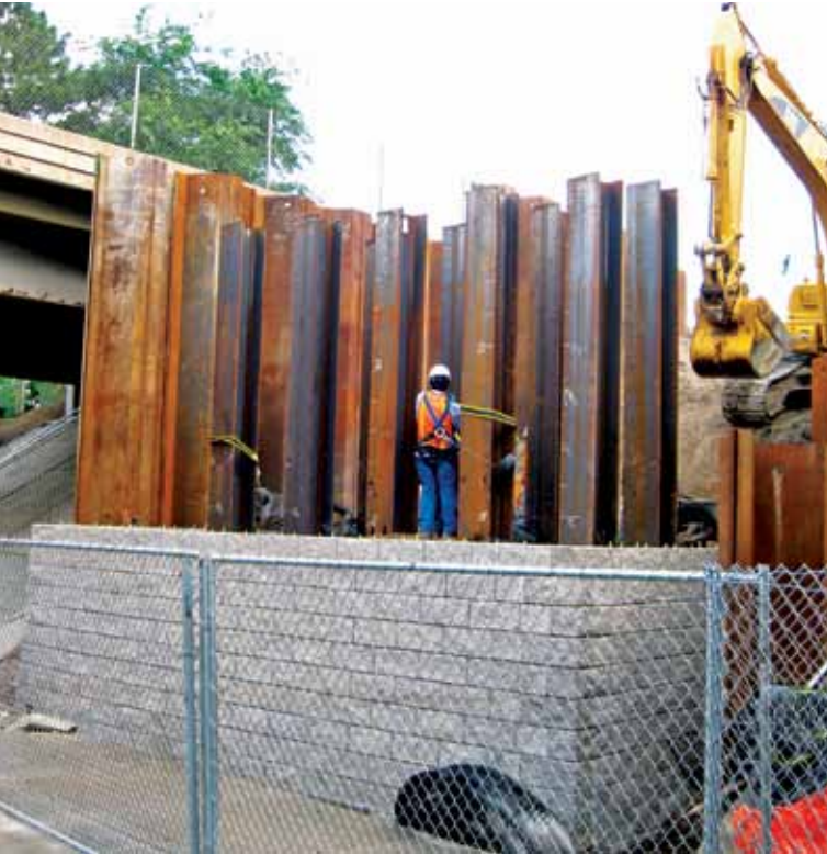
Abutment construction in between interstate bridges
