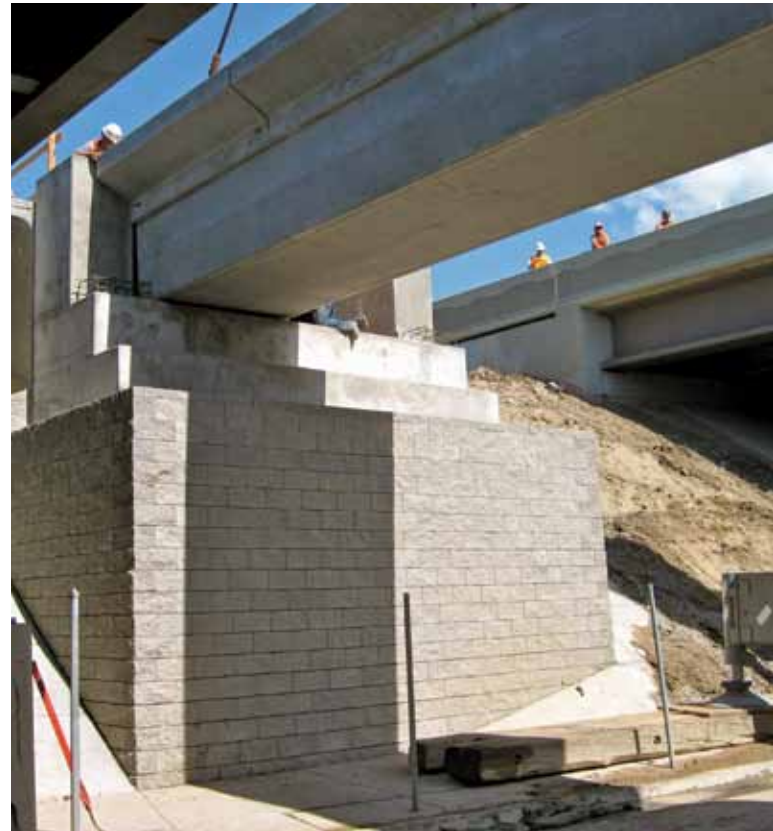
Completed Abutment with beams being set
