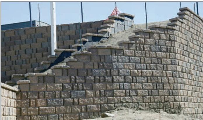
The Keystone Compac walls vary in total heights ranging from 28-30 feet with exposed heights nearing 20 feet. The site’s remote location and limited access points required that several efforts including wall installation, delivery, grading and foundation efforts occur simultaneously in a confined working area. As a result, extensive and daily coordination between the numerous contractors, engineering consultants, subcontractors and developer was required to meet a tight construction timeline.
