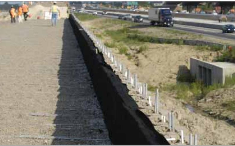
retaining walls approached heights of 40 feet in some locations, a cost-effective solution needed to be found that addressed these circumstances. KeySystem I was selected for its ability to deliver an economic and extremely strong structural solution for tall walls and extreme loading conditions.
