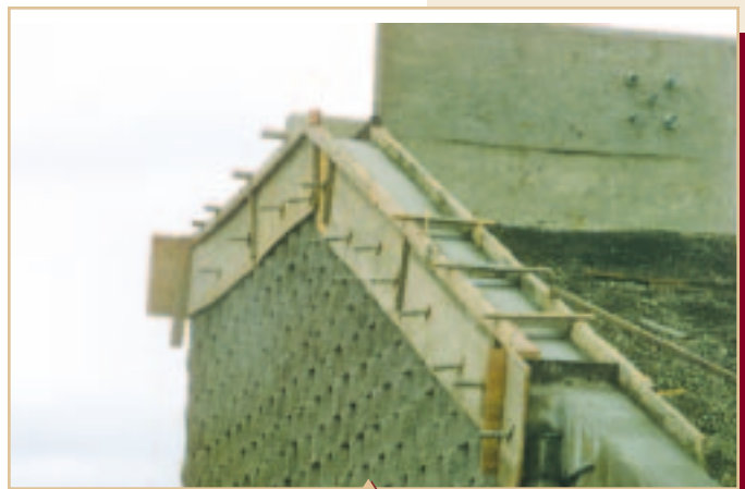
Forming of Site Poured Copings
