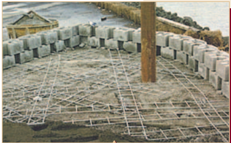
Steel Reinforcing Layout at Bridge Support Point
