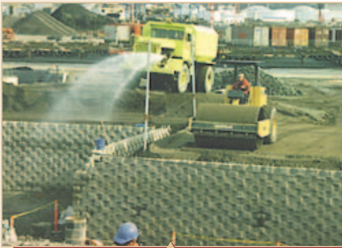
Select Granular Fill With Vibratory Compaction
