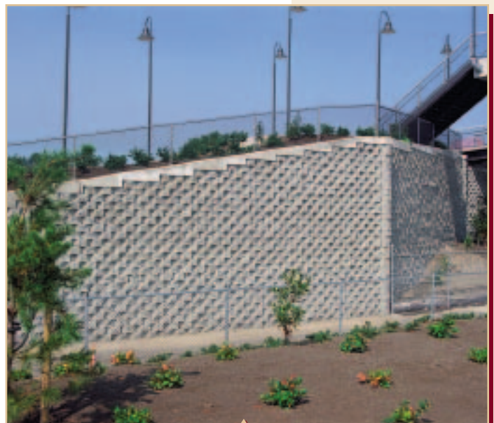
Pedestrian Ramp, Bridges and Overpass
