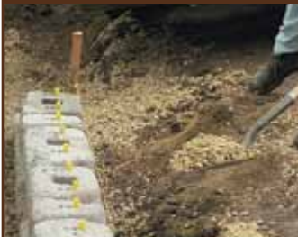
Avoid "stack bond" conditions where more than two courses create weak areas in the wall.
